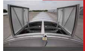
SMOKE VENTS IN CONTINUOUS ROOFLIGHTS
